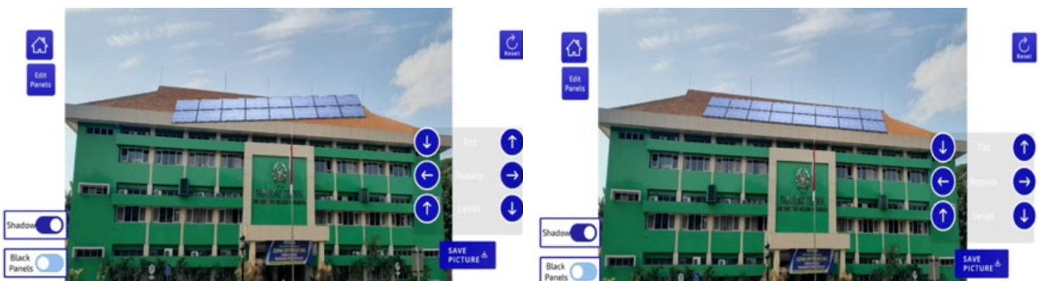
Fig. 5. Station PV system 16 panels in augmented reality
