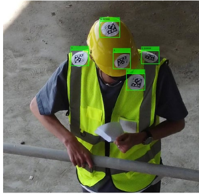
Fig. 5. DM tags on a worker's helmet and vest.
