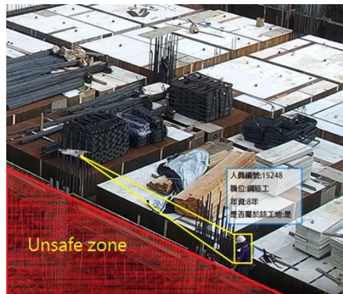
Fig. 3. UAV aerial inspection of an unsafe zone.
