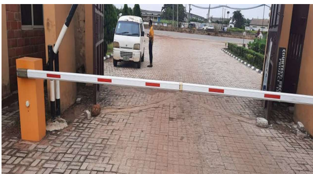
Fig. 3. The automatic boom barrier
