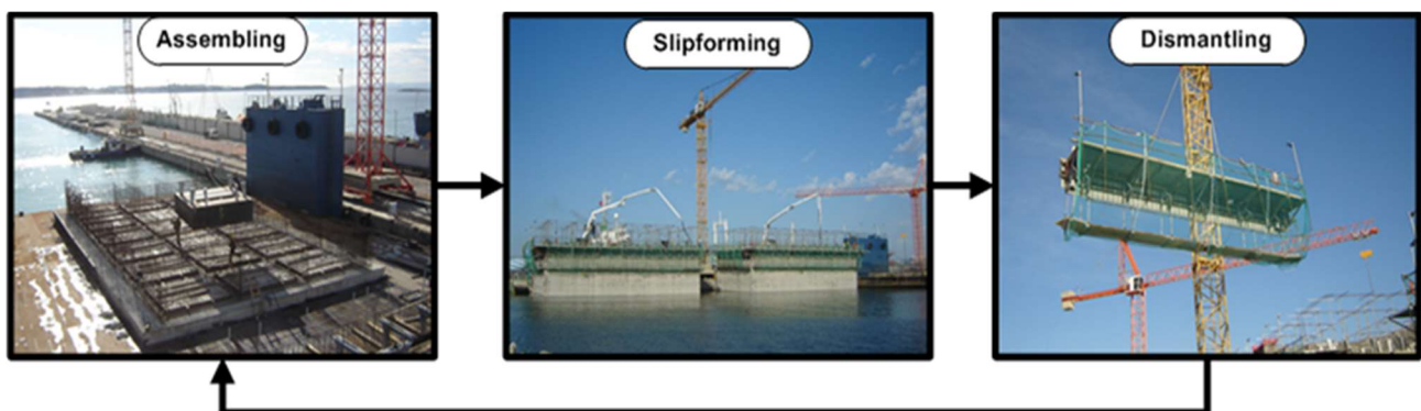
Fig. 3. Floating caisson production cycle (Source: Panas & Pantouvakis, 2018)
