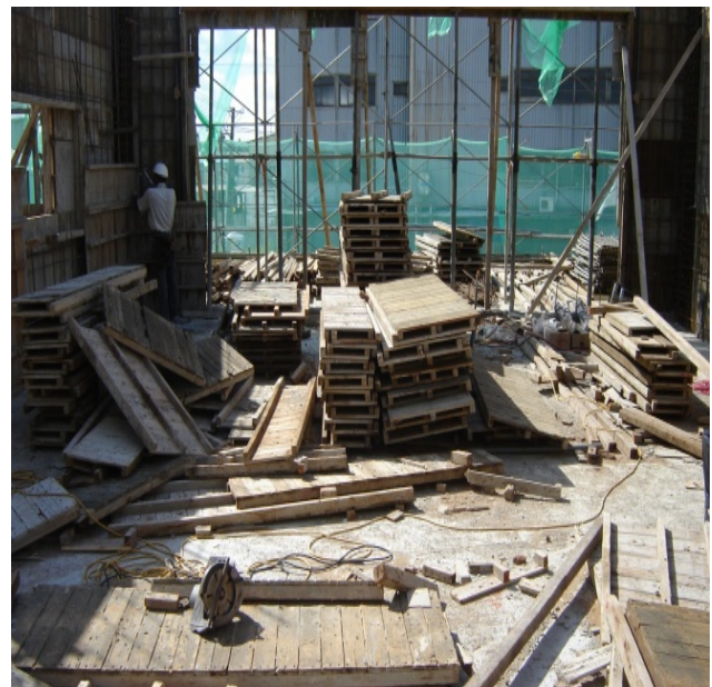
Fig. 3. Actual site of formwork implementation
