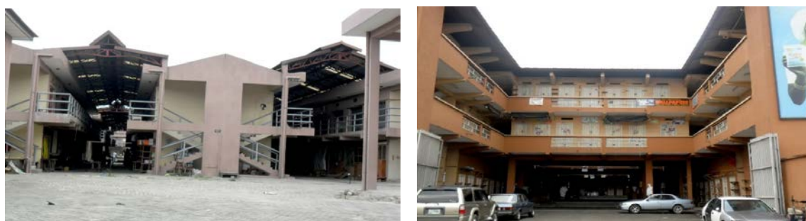
Figure 4. A Section of Remodelled Market South and North Respectively.
