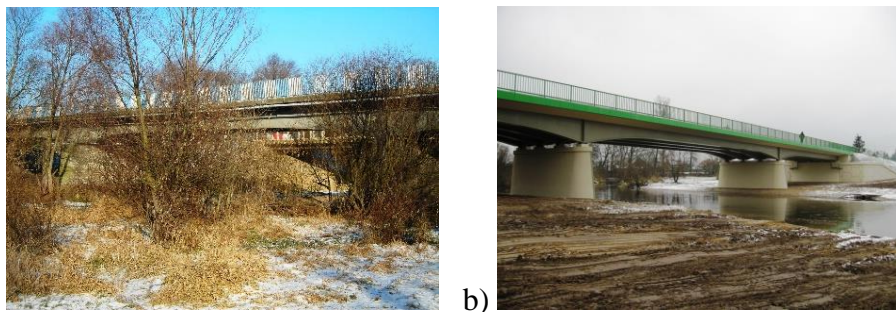
Figure 5. The bridge in Neple over the Bug River a) an old bridge b) the new one
