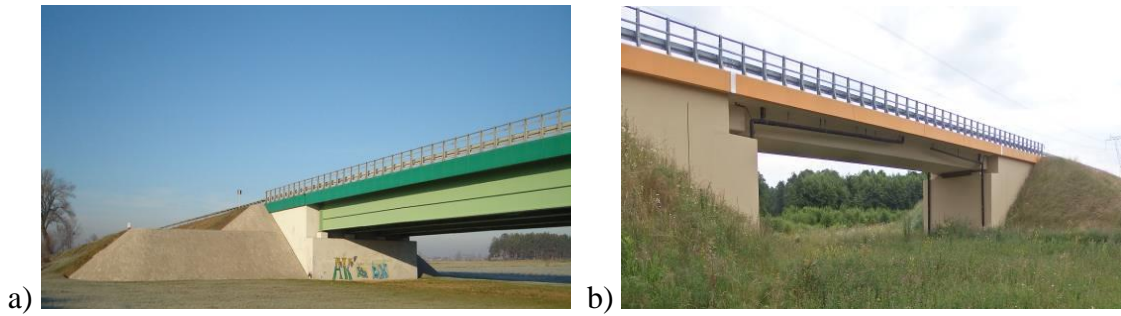
Figure 7. Bridge cone veneering a) natural grass b) concrete blocks
