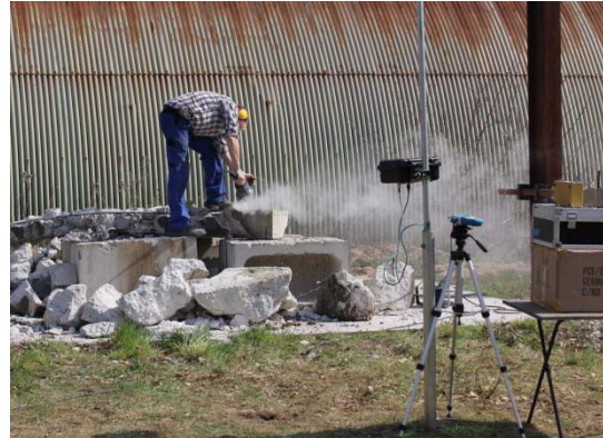
Figure 9. Fully equipped node used in a test
