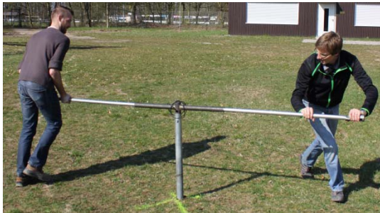
Figure 8. Turning an earth screw into the ground
