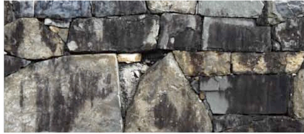
fig.18 The elevation of the stone wall
