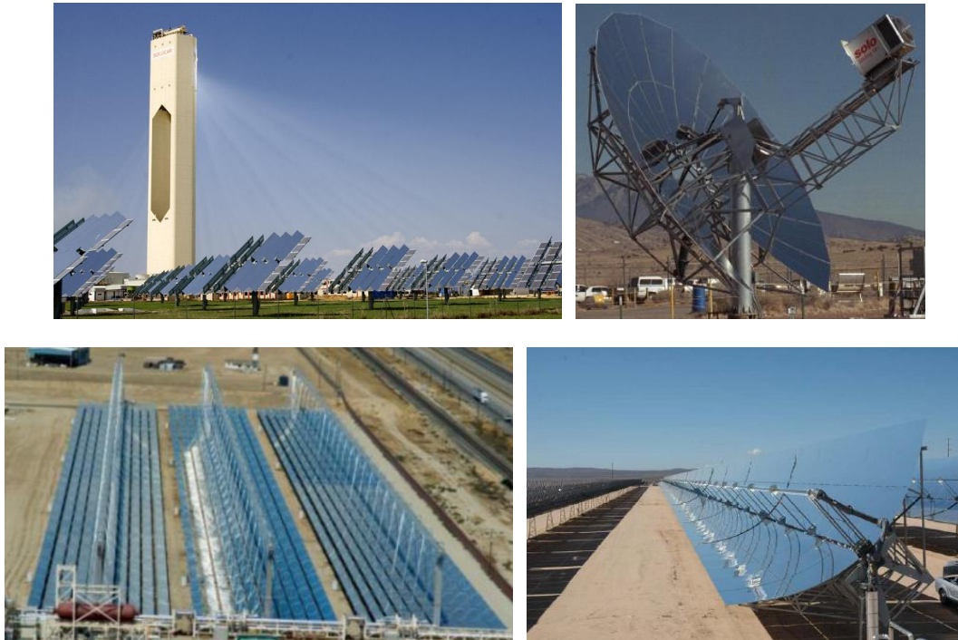
Figure 1: Four main commercial types of CSP plants: Abengoa Solar’s PS10 power tower, Seville, Spain (Top left) (Abengoa Solar, a, 2010); Flagsol parabolic troughs at Kramer Junction (SEGS V), California, USA (Bottom right) (Kearney, 2007); Sandia 10-kWe dish/String system (Top right) (Kearney, 2007); Linear Fresnel Reflectors at Kimberlina Solar power station, California, USA (Bottom left) (Areva Solar, 2010).
