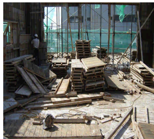
Figure 3. Actual Site of Formwork Implementation
