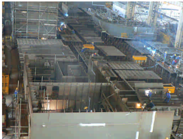
Figure 1. Block assembly in workshop
